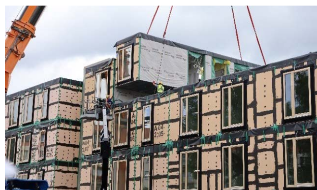
Fig. 7. [a] Design of the multi-family modular building in Mysłowice by DMDmodular; [b] Stage of modular building construction. Source: https://www.gov.pl/web/ncbr/ncbr-pokazalo-ekologiczny-budynek-w-myslowicach [access date: 13.11.2023]
