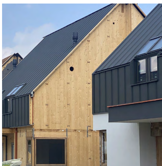
Fig. 3. Houses in Krakow constructed by Multicomfort using CLT, covered on the outside with thermal insulation panels and steel or plaster final finishes, protecting the timber structure from adverse weather conditions. This also reflects the social prejudice that it is better to live in a brick building than in a wooden house. Photo by the authors
