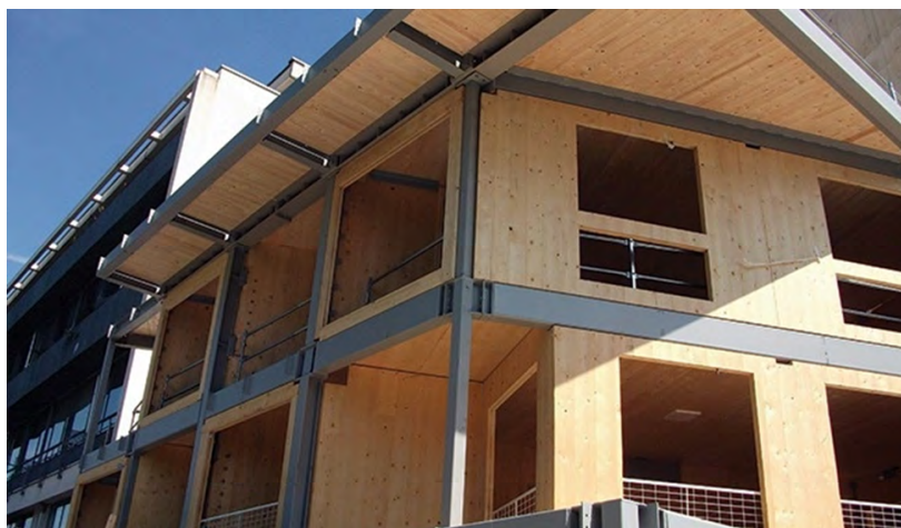
Fig. 4. An example of multistorey housing using CLT hybrid construction. Steel construction elements strengthen the structural skeleton of the building, while the CLT panels fill the wall and ceiling structure. Photo courtesy of Multicomfort
