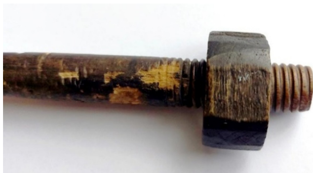
Fig. 2. Detail of the original wooden screw originally built in the structure of the Gliwice Radio Station tower (Fig.1)
