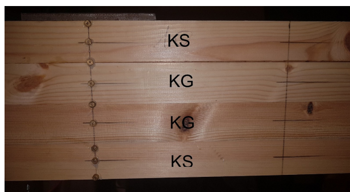
Fig. 1. Preparation of glued laminated beams for reinforcement
