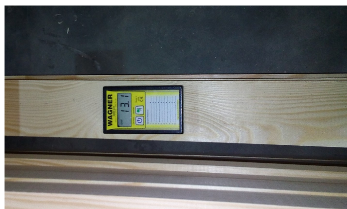
Fig. 2. Moisture measurement of an example beam (BEAMJ1-2)
